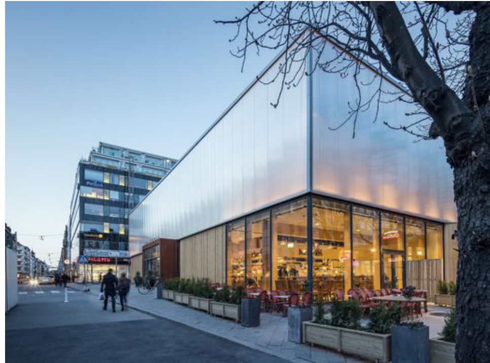
Stockholm temporary Market Hall
